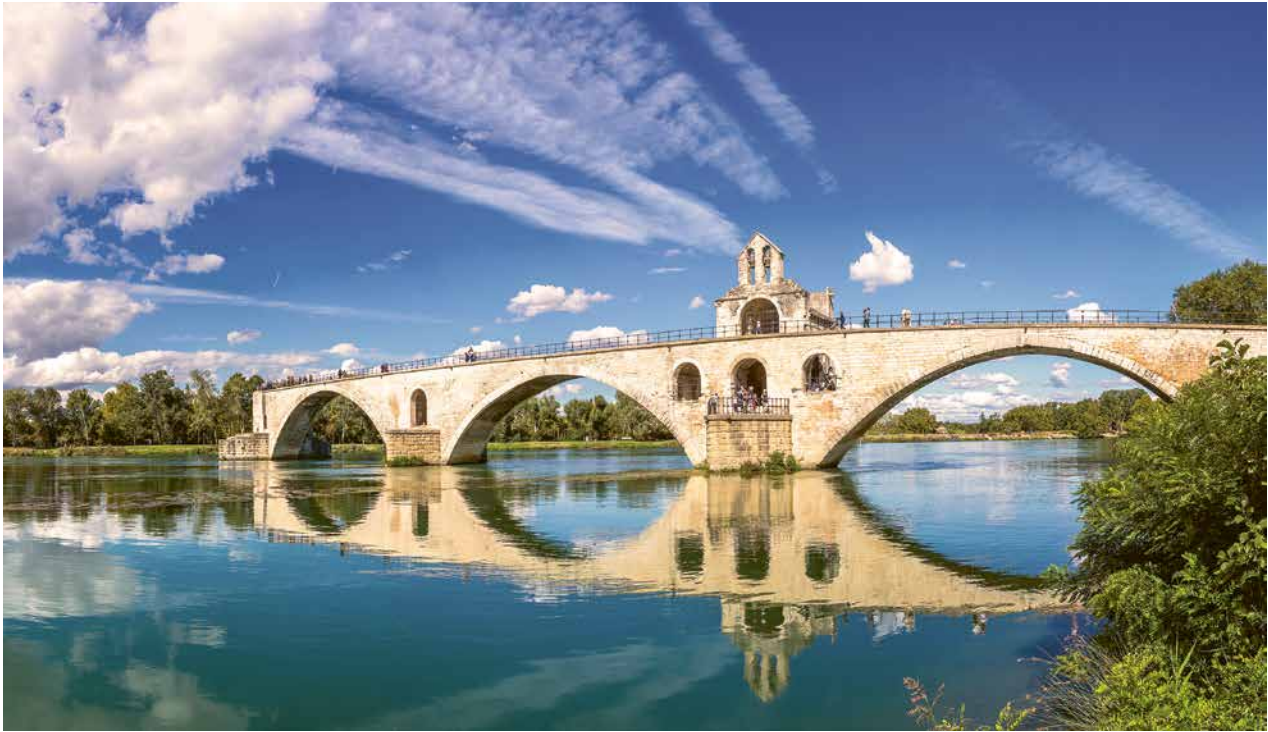
BRIDGE OF ST. BÉNÉZET
